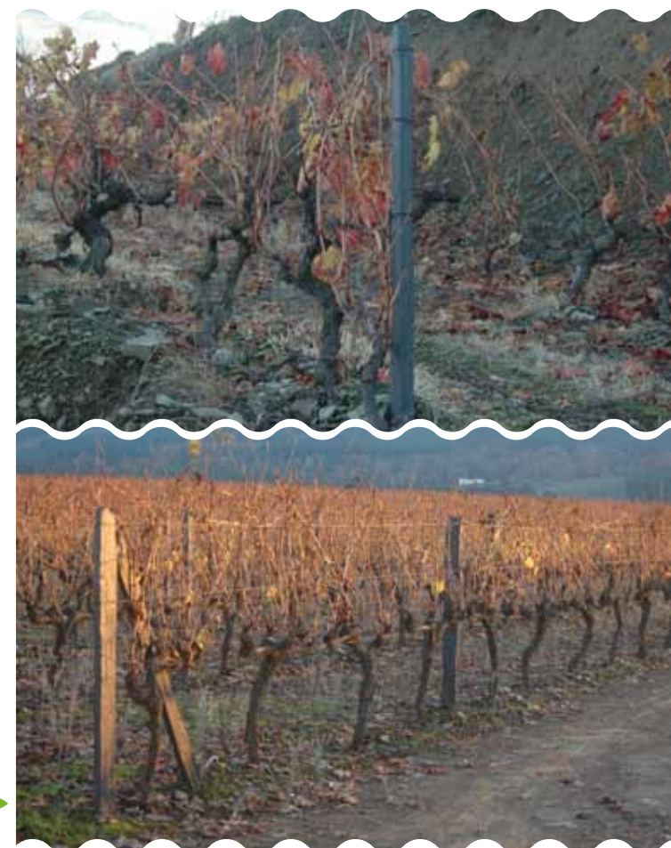
FIGURES 27A AND 27B - Incorrectly anchored end post (above); correctly anchored end post (below).
