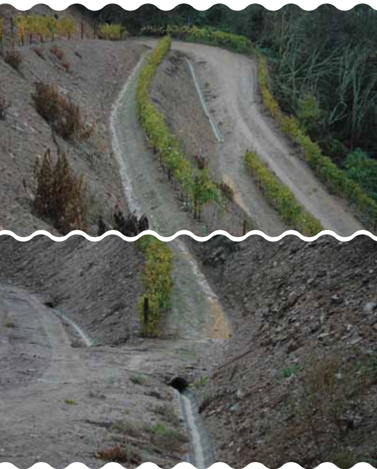
FIGURES 7A AND 7B - Half-pipe concrete drains placed along the access roads to single-row patamares that slant along their length and inwards to encourage the rainwater to run down the slope and into the drains, thus preventing it from creating ruts and cutting into the embankments (Quinta da Romaneira).
