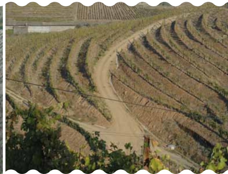
FIGURE 14 - Patamares with 1 row of vines. Surface water flows down the longitudinal slant of the patamares and along the open concrete pipe drains and culverts on the access roads.
