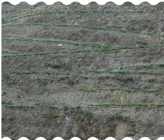
FIGURE 5 - Incorrectly formed patamares that, as they are not parallel to each other are supported by very irregular embankments in size and shape, will in turn create serious erosion problems and significantly increase the cost of the work in the vineyard.
