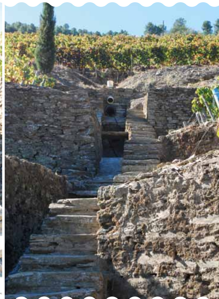
FIGURES 8A AND 8B - On the left, a correct drainage system along a water course dating back to pre-phylloxera times; on the right, the same system after it was destroyed upstream to make way for mechanized patamares, resulting in serious erosion to the embankments.
